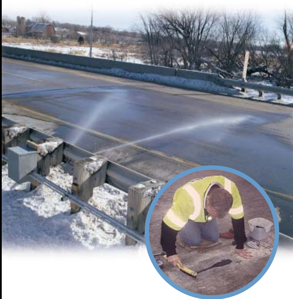
Pavement sensor installation.
