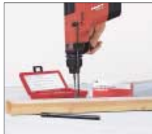
Drill a hole 1/2" deeper than the required screw penetration.
